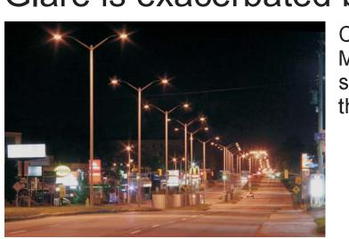
Comparison of FCO luminaires (near field) and non-FCO luminaires in the distance. Maximum illumination level was about 17-lx. Unregulated commercial signs cause significant distracting clutter for motorists - especially the flashing or animated signs that delay driver reaction times.
